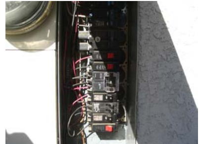
Electrical panel in good order
